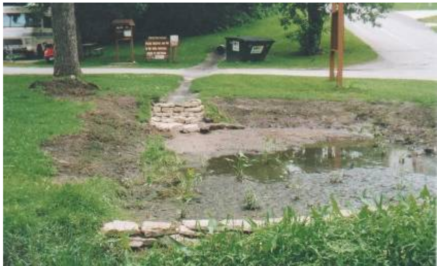
Stormwater detention basin in Lanesboro city park traps sediments before they enter the fishing ponds.
