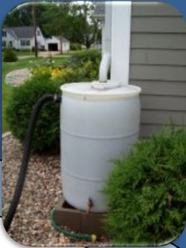
A rain barrel is a rainwater collection system that stores rooftop runoff for use later to water lawns and gardens.
