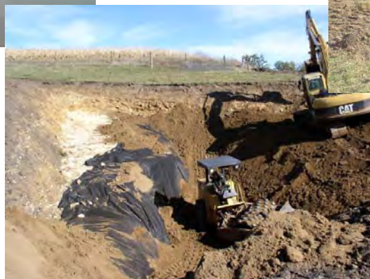
Sinkhole is dug out to the "eye", filled with rock, lined with fabric and covered with soil
