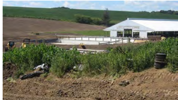
Newburg Twp Feedlot AFTER
