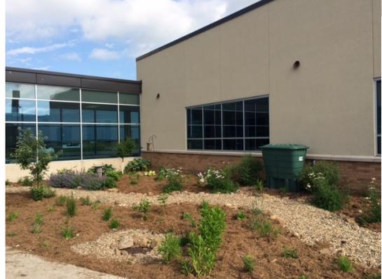
Above: In the courtyard of Kingsland Public School, existing turf grass was replaced with a rain garden and cisterns to collect roof-top run-off. This project will reduce run-off by over 30,000 gallons per year.
