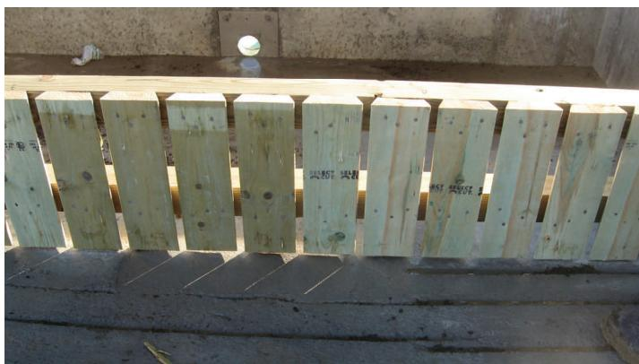
Example of a picket dam used to separate the solids in the manure from the liquids; solids are scraped from the lot and land applied; liquids are filtered in a grass filter strip
