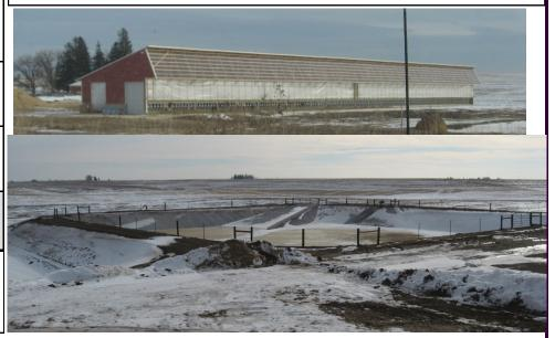
After: Relocation of feedlot site with total confinement barn with waste transfer system to manure storage structure.
