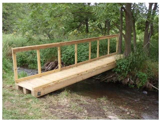
This swing-away bridge is secured by cables on the far side of the river and is resting unattached on opposite bank.
